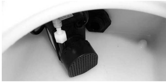
Pump placement in water tank.
