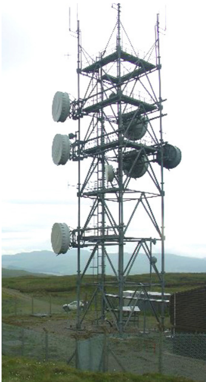
Figure 6a. Microwave repeater showing multiple co-located antennas. 3
